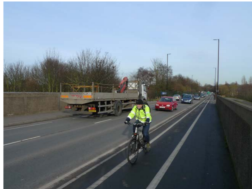
Existing Severus bridge deck view
