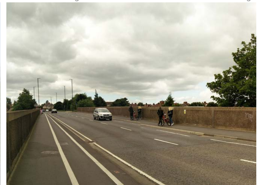
Existing Severus bridge deck view
