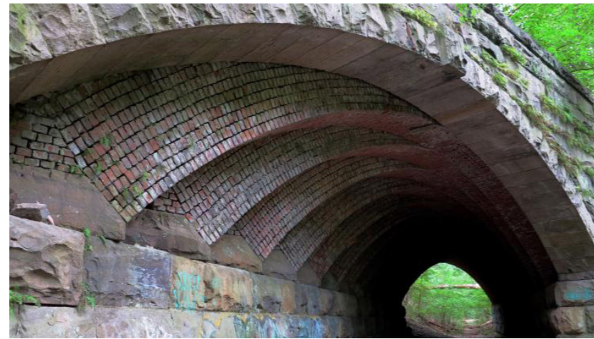
Skewed brick bridge
