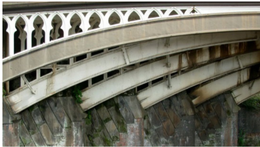
Skewed steel bridge
