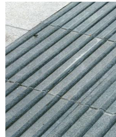
P4. Concrete corduroy paving
