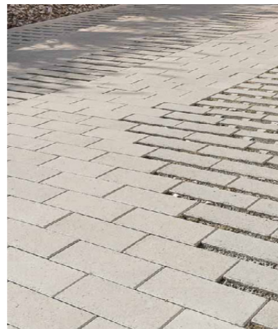
P3. Concrete permeable block paving
