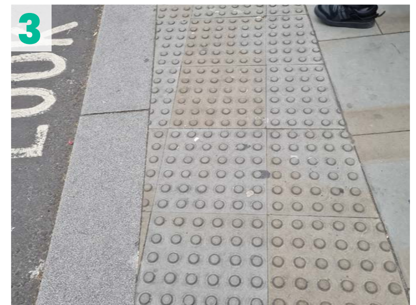
Tactile paving at pedestrian crossing points
